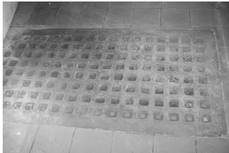
Figure 3: Example of an illuminating tile made of concrete and glass; (S. Wermiel, photographer)
